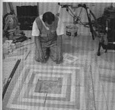
Pawel made the whole frame first and cut out the star afterwards.
