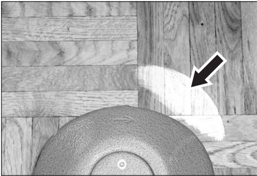
Fig. 65 Improper adjustment of the guide rollers: The sanding zone of the machine is too much to the right .
