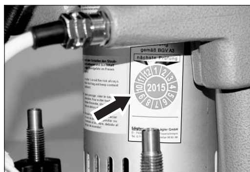
Fig. 70 The inspection label on the motor housing confirms the electrical and mechanical safety of the machine.
